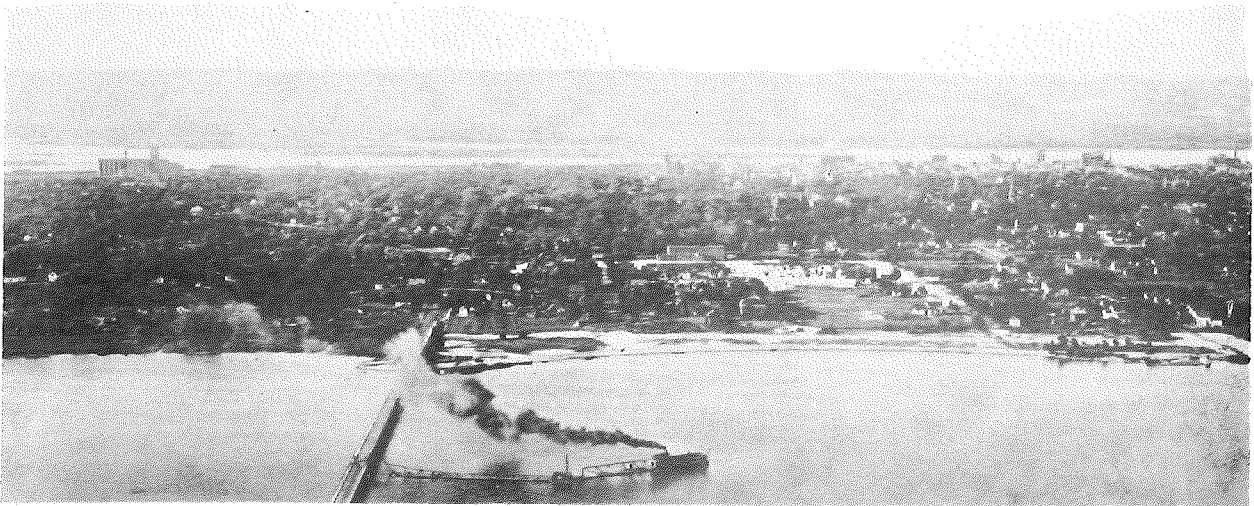
Fig. 3-6 Construction of Lake Park, Maxwell Field and Huff Street Causeway with soil dredged from Lake Winona in 1913. Photo reference same as Fig. 3-5.
