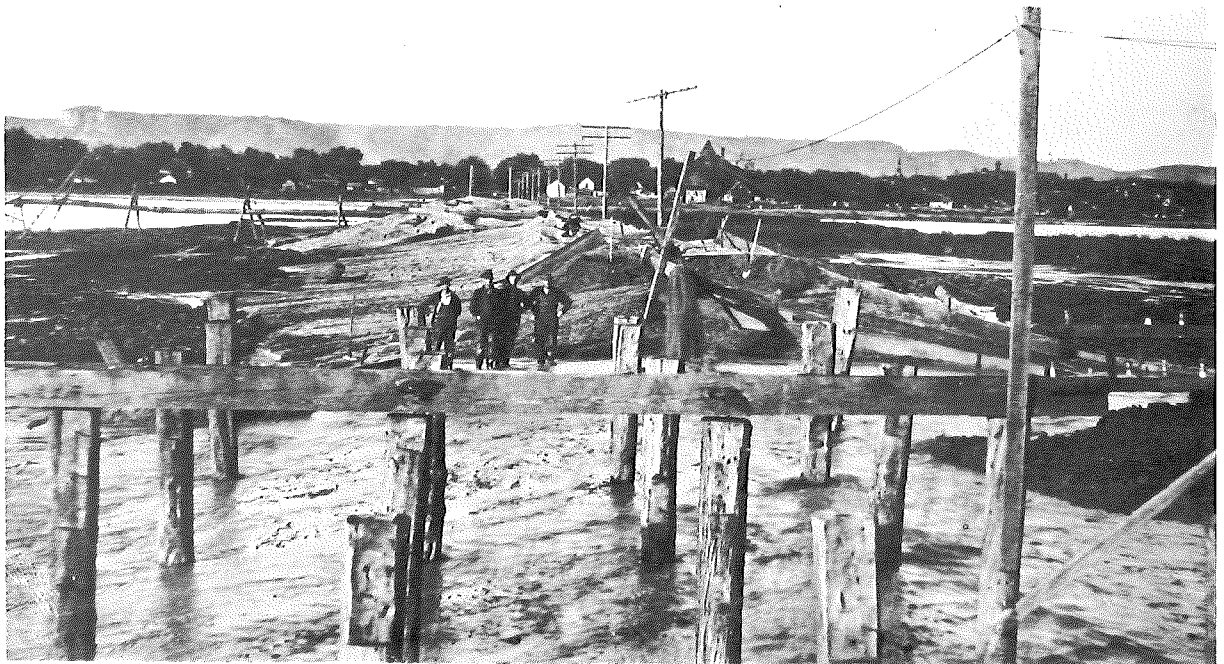
Fig. 3-7 Construction of Huff Street Causeway by dredging in 1913. Photo reference same as Fig. 3-5.
