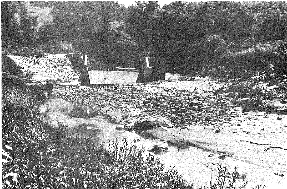
Fig. 3-12 Severe streambank erosion along Gilmore Creek caused by flooding during the 1930's. View is toward Knopp Valley from St. Mary's College campus. Note wing dams. 1938 USDA photo.
