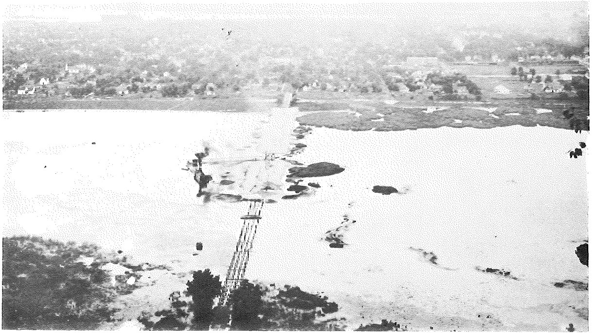
Fig. 3-7 Construction of Huff Street Causeway by dredging in 1913. Photo reference same as Fig. 3-5.
