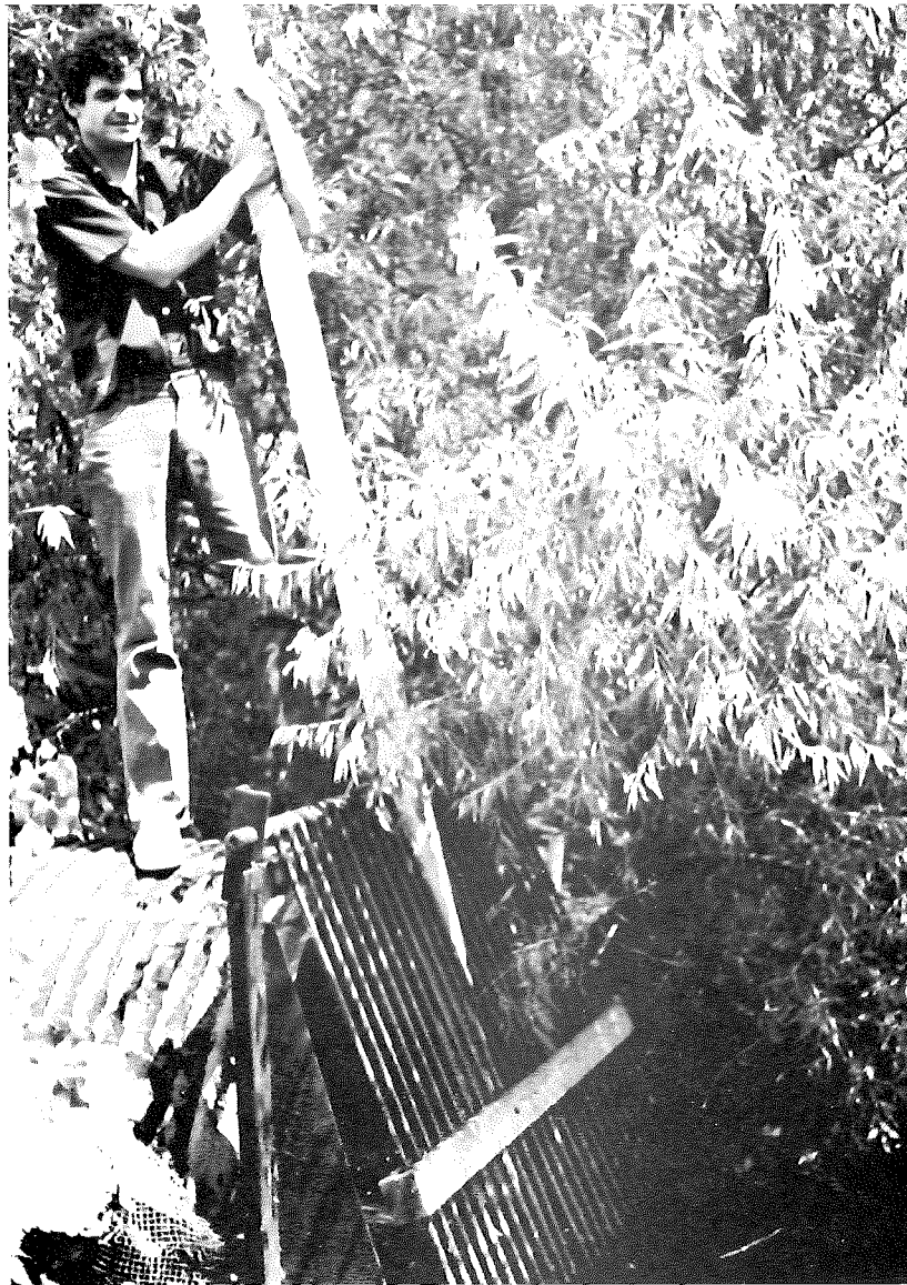
Figure 11-10. A carp barrier at the downstream end of County Ditch No. 3 prevents carp and buffalo from swimming upstream into Boller Lake to spawn.
